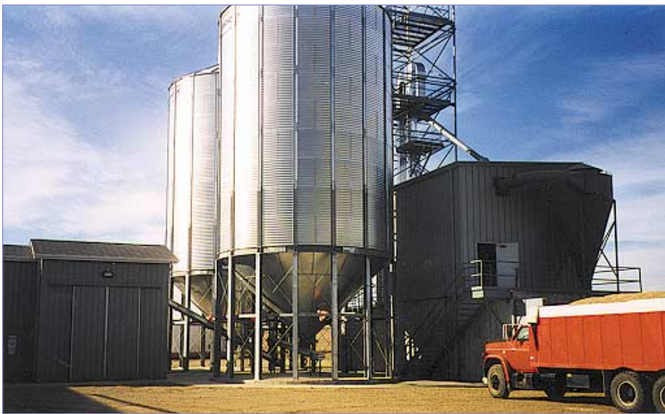
The new plant — owned by soybean and canola farmers — is producing sustainable, non-toxic and biodegradable crankcase oil and lubricants. USDA Photo by Bobbie Morrison
