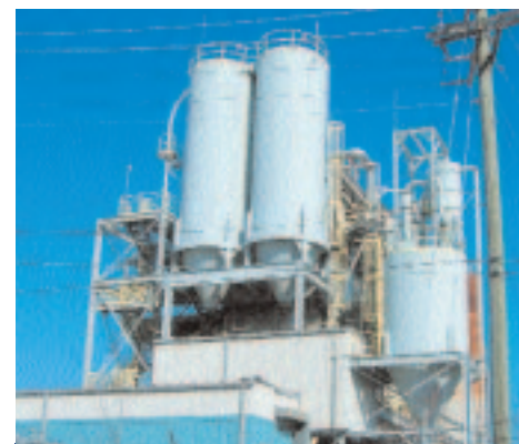
Electrical plants in Georgia (above) and Kansas are being disassembled and moved to Carnesville, Ga., where the parts will be used to build Plant Carl. Photo by Billy Jones
