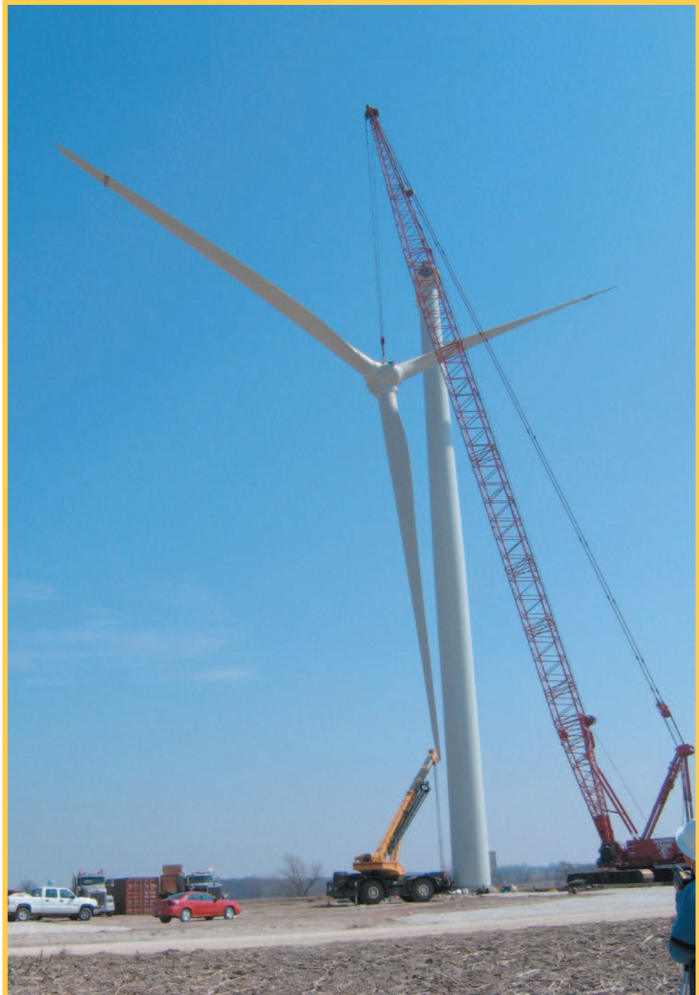
Many parts of the nation previously thought to lack wind resources can now generate wind power, thanks to advances in turbine technology. This turbine was recently erected by the Illinois Rural Electric Cooperative (IREC). Photo courtesy IREC
