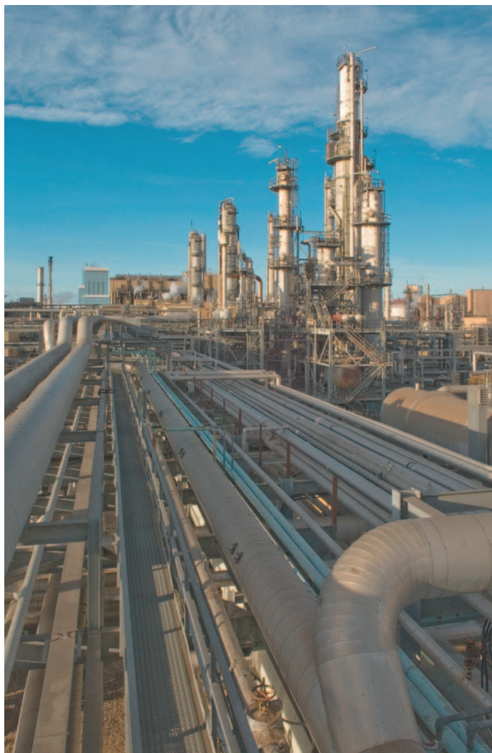
The Great Plains Synfuel plant, run by a Basin Electric subsidiary, converts dirty, low-quality lignite coal into clean-burning natural gas. The carbon dioxide generated by the conversion is recovered and injected into Canadian oil fields, forcing out petroleum that would otherwise be inaccessible.
