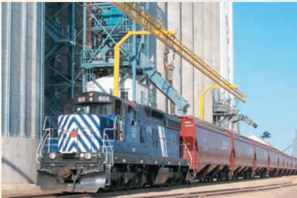
South Dakota Wheat Growers' (SDWG) wheat segregating facility in McLaughlin loads its first train. The concrete silos were already there, but the steel loading structures and new tracks were recently added. Photo courtesy SDWG
