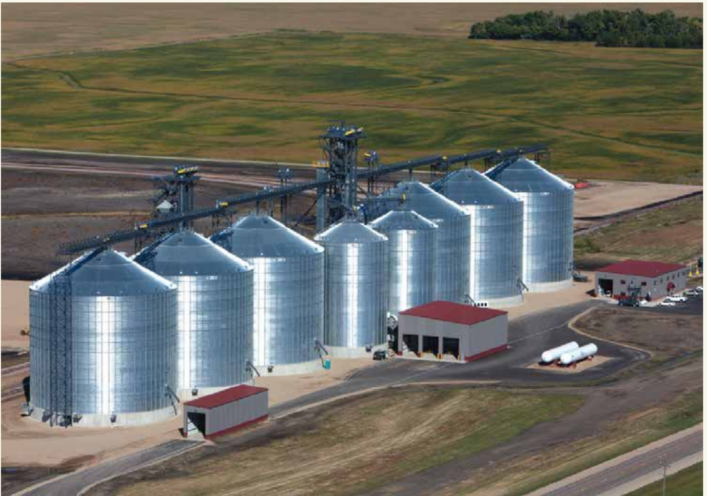
Wheaton-Dumont Cooperative (WDC) finished work on its Graceville Grain Terminal, near Graceville, Minn., in September 2013. The facility has upright steel-storage capacity of 5 million bushels, with a temporary capacity of 2.8 million bushels. The fully automated facility can receive grain at 60,000 bushels per hour. It is served by a loop track that can accommodate 120 railcars and loads at 80,000 bushels per hour. Photo courtesy WDC
