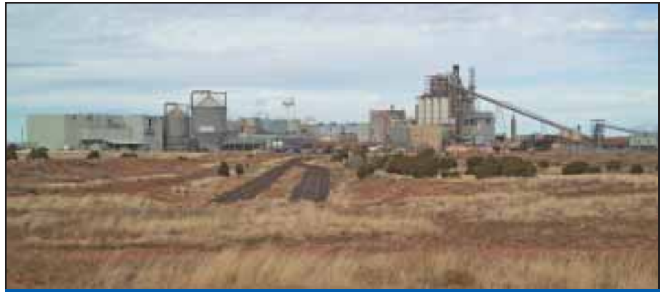
A biomass powerplant is being built adjacent to this papermill in Arizona. The biomass plant will produce 20 megawatts of electricity from mill and forest wastes.
