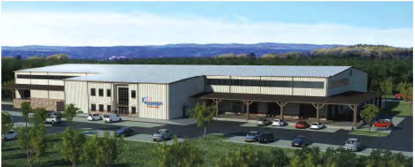
Second Harvest's new, 65,000-square-foot regional food distribution center in Thomasville, Ga., benefitted from $5.2 million in funding from USDA Rural Development.
