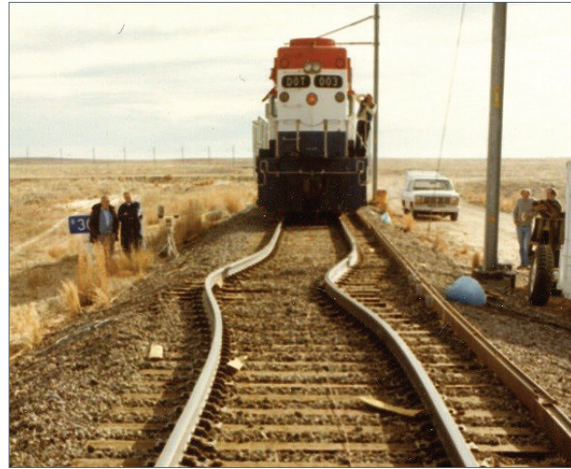
Figure 2-9. Rail Thermal Misalignment 135
