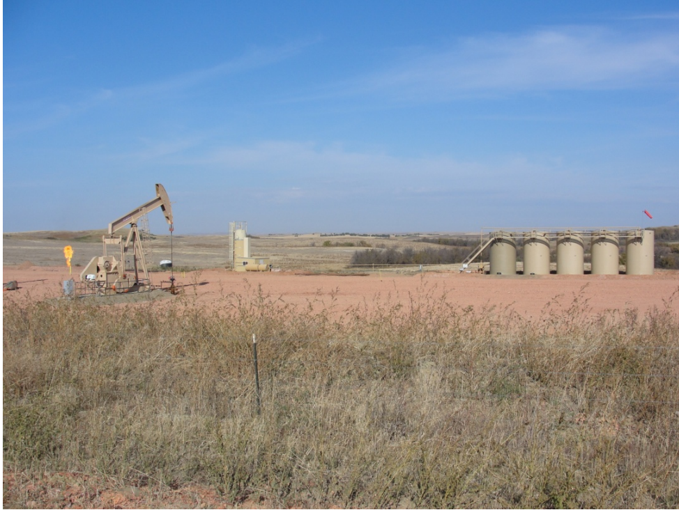
Figure 3-7: Typical Oil Well Pad Site
