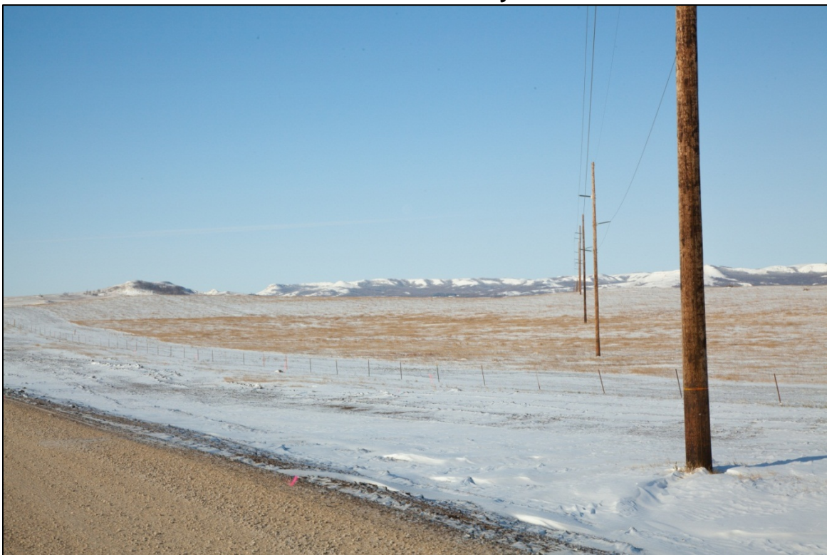
Figure 3-8: 115-Kv Transmission Line Near the Killdeer Mountain Battlefield Study Area
