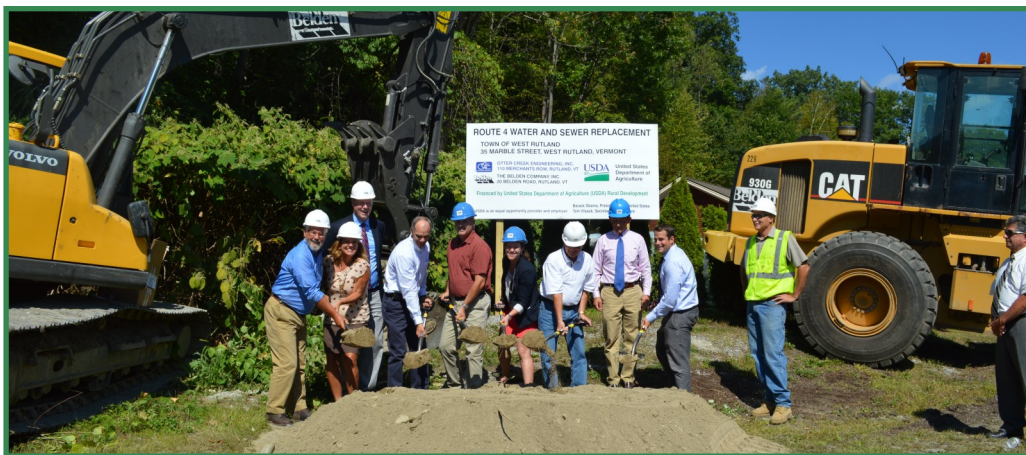
The Town of West Rutland celebrates their new water and sewer main extension. West Rutland received over $2 million in loans and grants from USDA Rural Development to help bring adequate water services to its businesses and residents.
