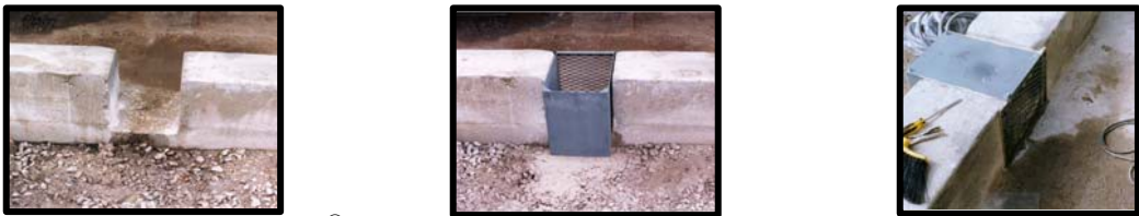
Figure 6-9: Imbiber Beads Gravity-Flow Drain Protection System—Curb Application
