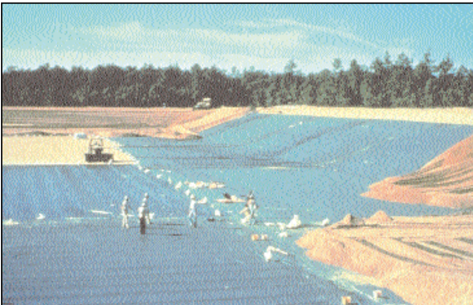
The membrane sealing the bottom of this landfill will prevent garbage from causing groundwater contamination. With the addition of a second membrane sealing the top of the finished landfill, the methane gas generated by the decay of refuse can be recovered and burned to produce electric power. Photos courtesy National Renewable Energy Laboratory
