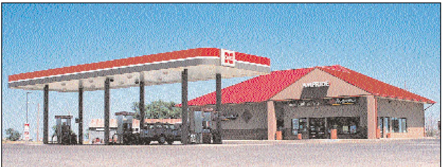
This CENEX/AMPRIDE C-store is one of two such operations generating new income for the Crosby County Fuel Association in Texas. Photos by Lynette Cockerell, courtesy PCCA
