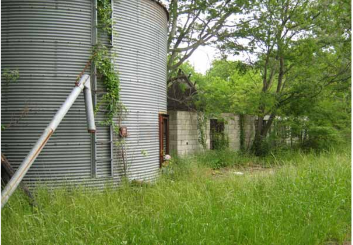
Figure 106. Nonhistoric farm complex in the eastern section of the survey area. View east.
