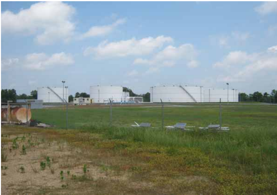
Figure 20. TEPPCO Boligee Intermodel Terminal within the southern boundaries of Site 1Gr31. View west.
