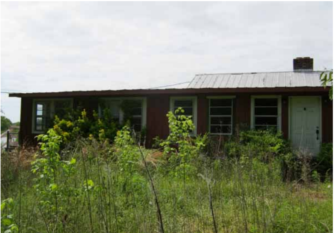
Figure 109. Circa 1960s nonhistoric hunting lodge in the east section of the survey area. View south.
