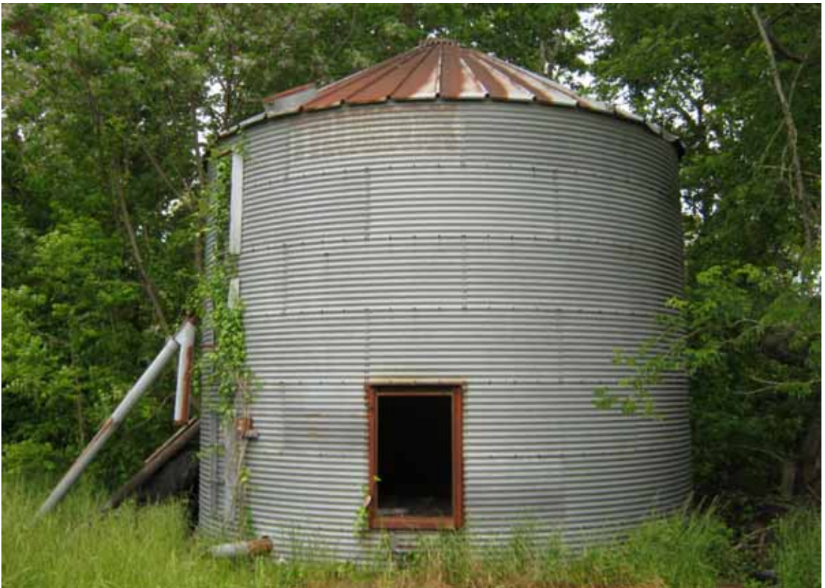
Figure 107. A grain silo associated with a deteriorated farm complex. View northwest.
