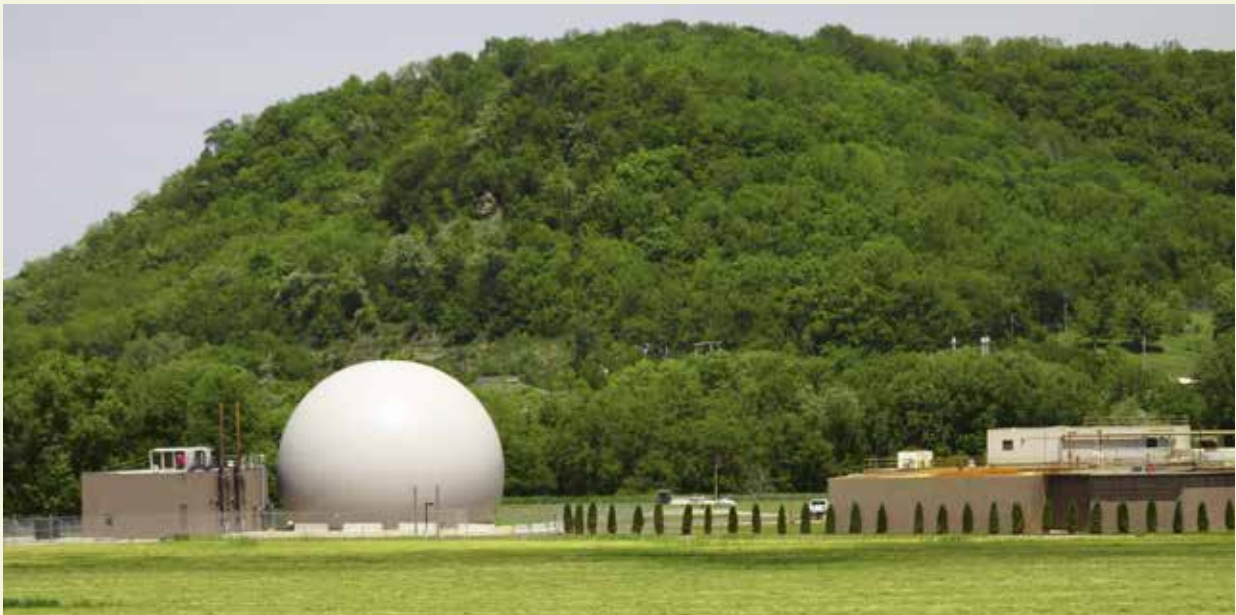
This industrial wastewater treatment facility at Richland Center, Wis., captures methane produced in anaerobic processes. The methane gas fuels an engine-driven electrical generator that creates electricity, which is sold to a local utility. Photo courtesy Foremost Farms
