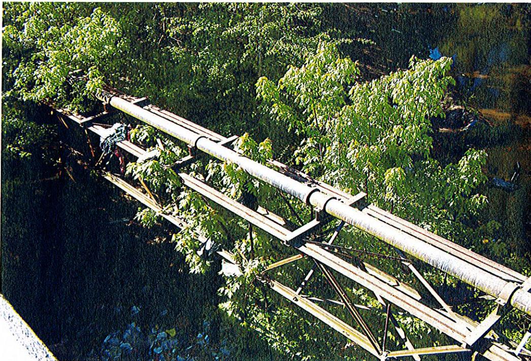
Photograph 8 - View of leaking sanitary sewer line spanning Brush Creek. Viewed from
