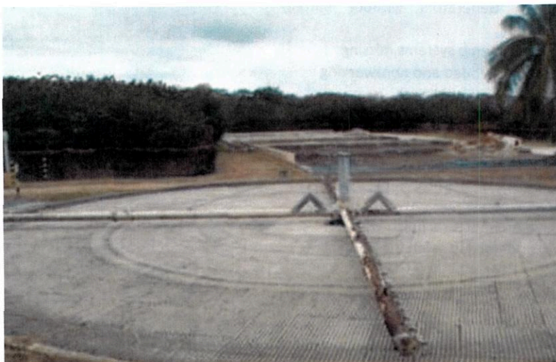
Figure 11 Trickling Filter at Forrestal WWTP
