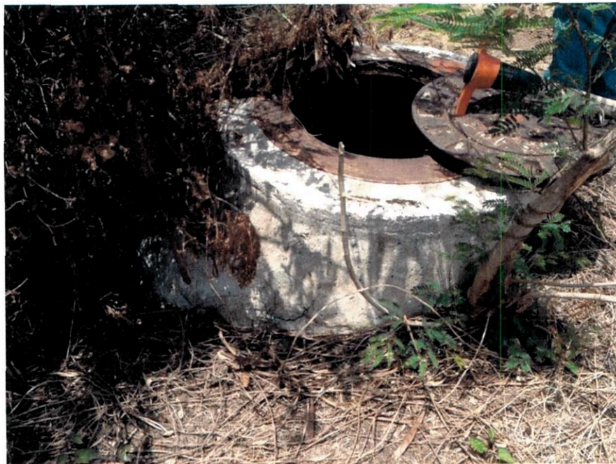
Figure 3 Typical gravity sewer system manhole
