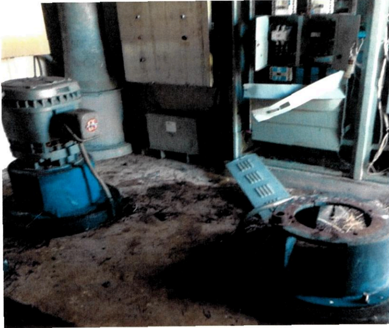
Figure 10 Lift Station 2382 Interior View
