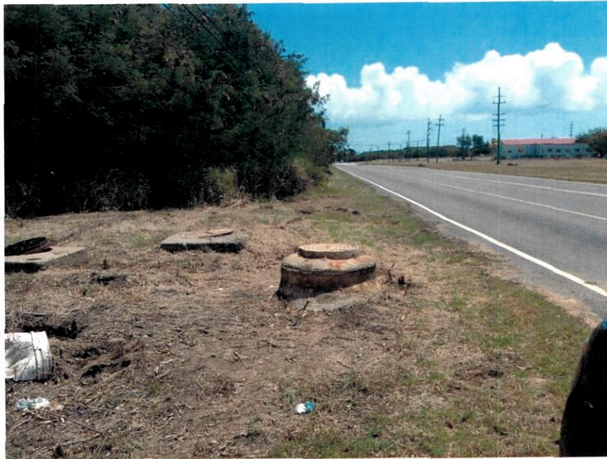
Figure 2 Typical gravity sewer system manholes
