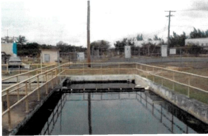
Figure 12 Primary Clarifier at Forrestal WWTP
