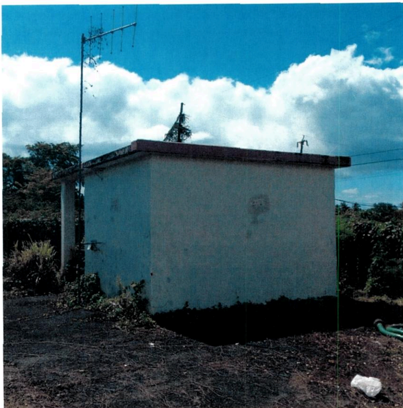
Figure 9 Lift Station 2382 Exterior View
