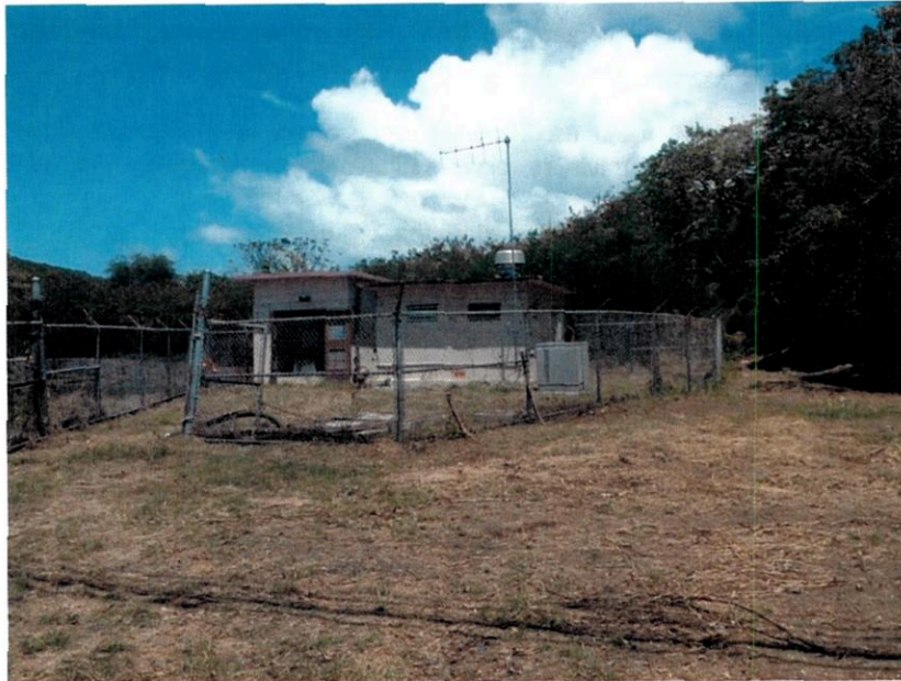
Figure 5 Lift Station 39 Exterior View
