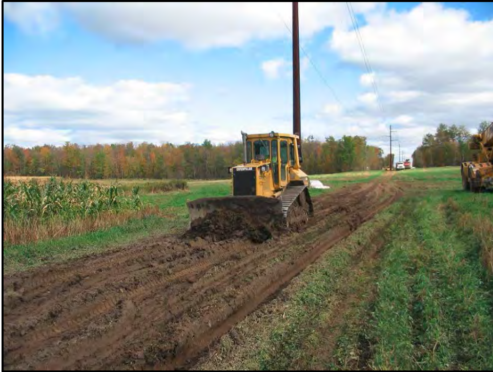
Figure D-2. Ruts being smoothed with blade.
