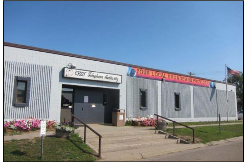
The first tribally-owned telephone company in the United States, CRST Telephone Authority continues advancing its nearly 60 year telecommunications history by investing in fiber optic upgrades.
