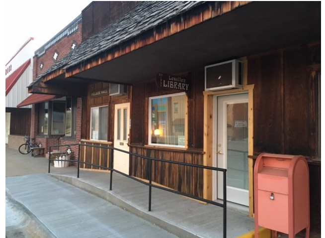
Ramp provides library accessibility for all patrons.
