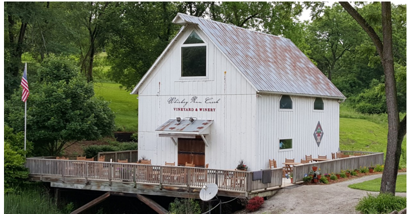
100 year old barn relocated spanning Whiskey Run Creek.
