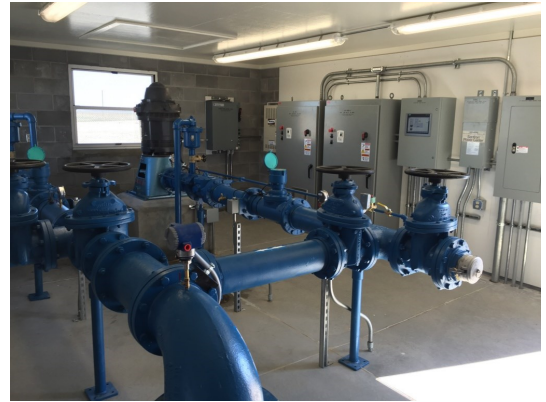
A look inside the well house.
