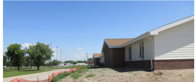
Expansion under construction.
