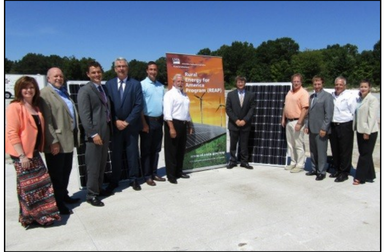
The USDA Rural Development REAP grant assisted Scott Black Inc. with funds needed to install a solar array in Humboldt, Tenn.
