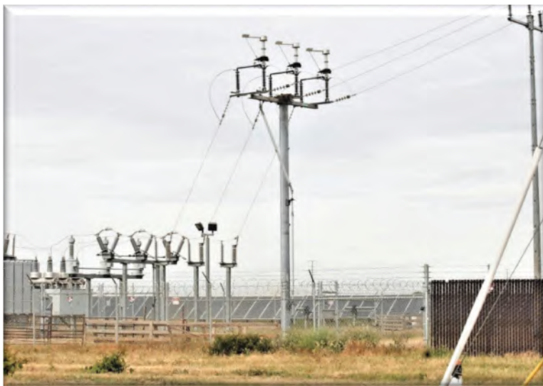
Plate 4. Swainson's hawk nest in the Kammerer substation, 2021.
