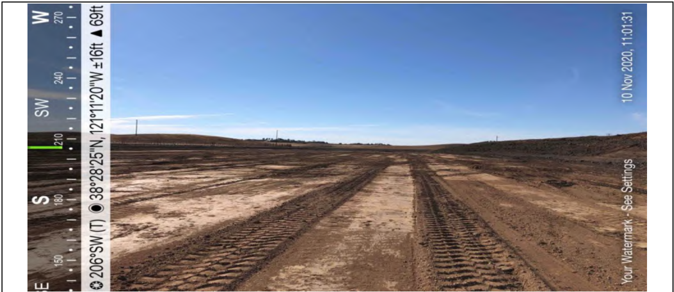
Photo 5: Grading within the PSA during the October/November field surveys.
