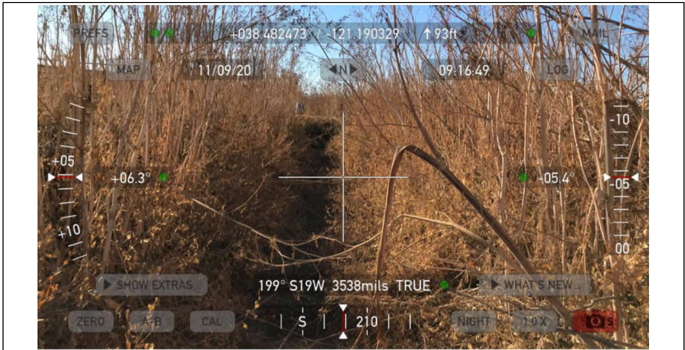
Photo 7: Representative photo of Ditch-02, which was inundated at the time of the October/November field survey and contained mostly upland vegetation.
