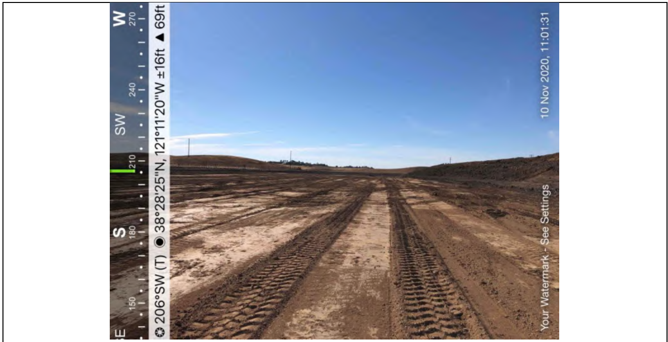
Photo 5: Pond-03 (pictured) was actively being graded during the October/November field surveys.
