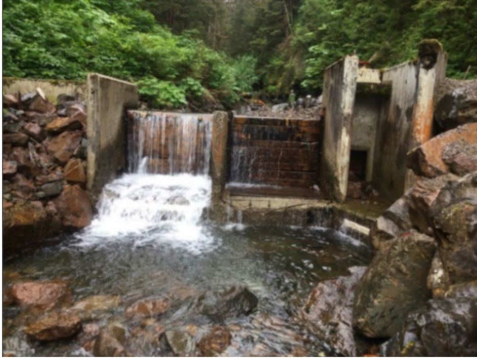
Figure 6 City of Hoonah water supply intake and location of the proposed hydroelectric facility tailrace. Photo taken August 9, 2023 (ADF&G 2023).
