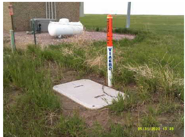
Photo #18 View of cable on the northeast portion of the site.
