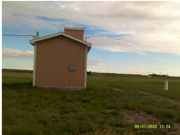
Photo #1 View of a well house (#1) on the northeast corner of the site.
