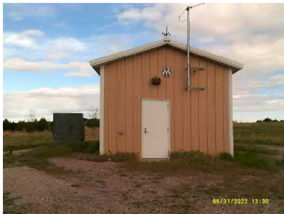
Photo #9 View of wellhouse (#3) with pad mounted transformer, looking west.
