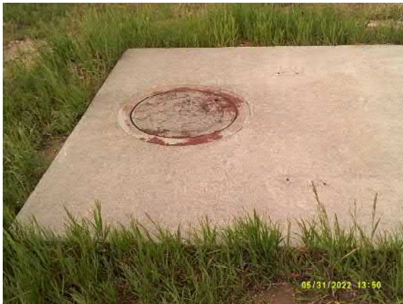
Photo #21 View of well on northeast corner of site.
