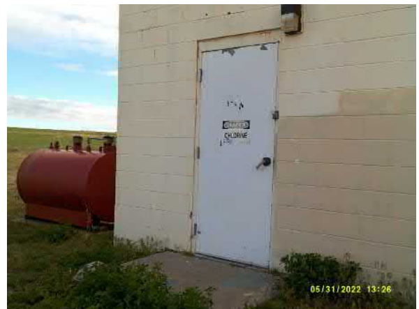
Photo #6 View of signage on door of well house.
