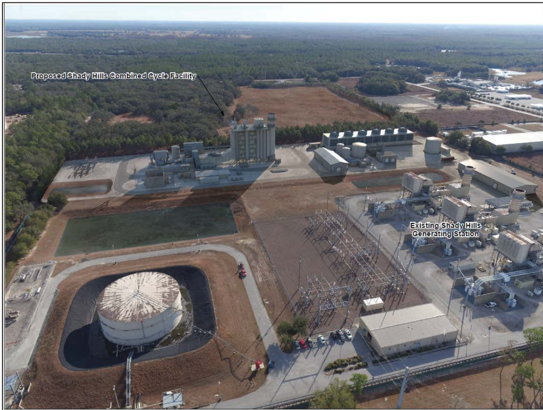
Figure 3. Conceptual Rendering of SHCCF and the existing Shady Hills Generating Station Looking East (SHEC SHCCF SCA Figure 1.1-2)
