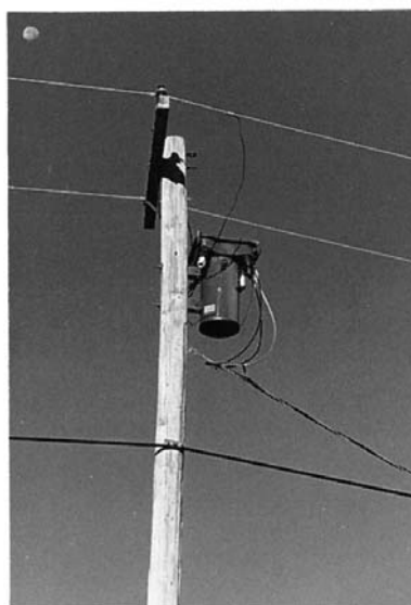
FIG. X1.3 Typical Pole-Mounted Transformer
