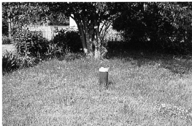
NOTE 1—Approximately 8-in. (203-mm) diameter. FIG. X1.10 Water Supply Well for Residential Property
