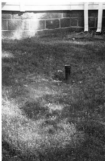
NOTE 1—Approximately 2½-in. (64-mm) diameter with screw cap. FIG. X1.9 Fill Pipe for Residential Underground Fuel Oil Storage Tank
