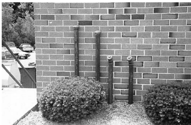
FIG. X1.7 Two Fill and Vent Pipes Leading to Two Underground Storage Tanks
