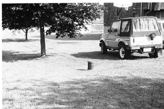
NOTE 1—Approximately 8-in. (203-mm) diameter FIG. X1.11 Water Supply Well for Residential Property
