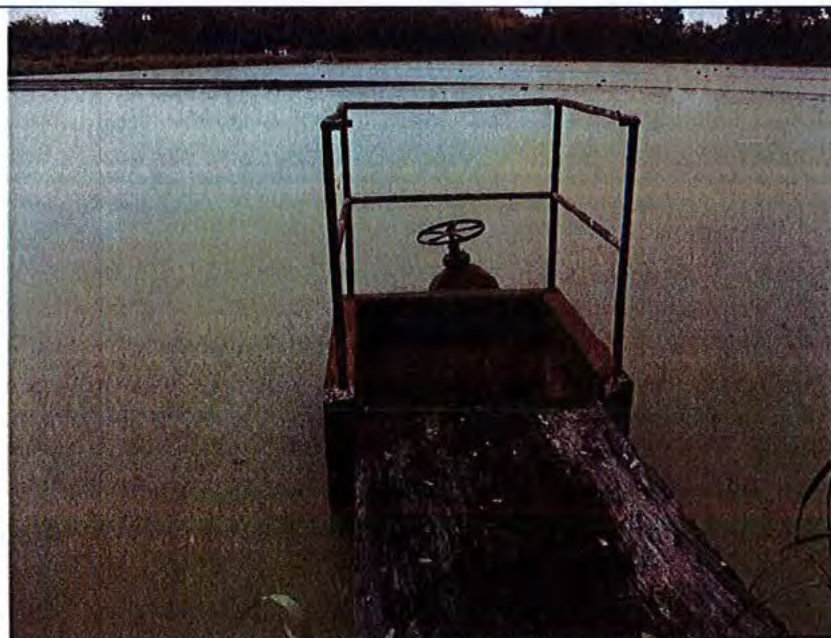
Emergency overflow outfall constructed at a former discharge point. Discharge was unpermitted and went to Cottonwood Creek. Heavy duckweed was observed in third cell in the series at the discharge point.
