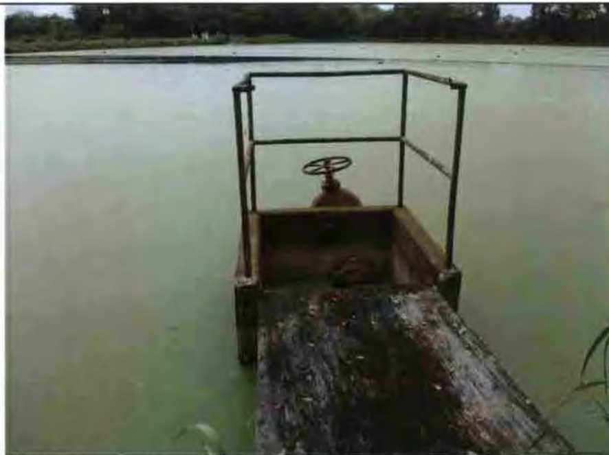
Emergency overflow outfall constructed at a former discharge point. Discharge was unpermitted and went to Cottonwood Creek. Heavy duckweed was observed in third cell in the series at the discharge point.
