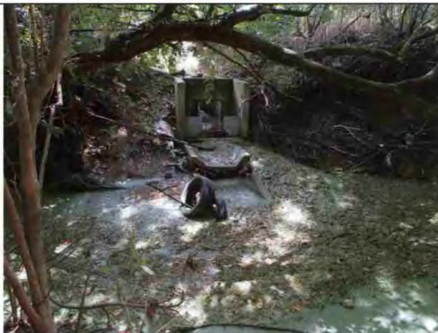
Heavy duckweed observed in Cottonwood Creek at unpermitted emergency overflow outfall from third cell of lagoon.
