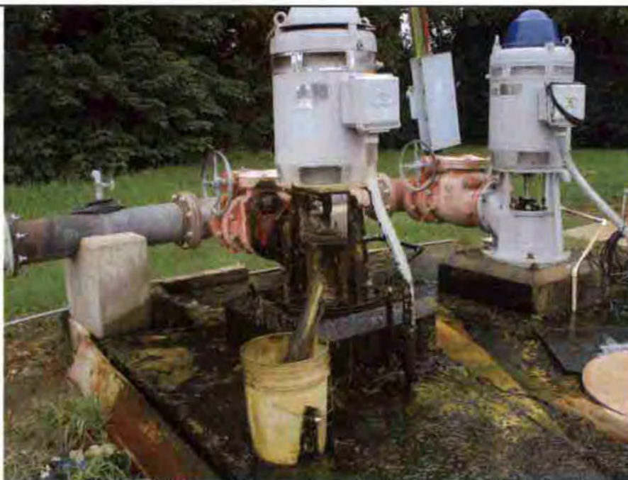
Two effluent pumps to facility's sprayfield. Heavy leak was observed at the left pump above yellow bucket. Water was ground absorbed.
