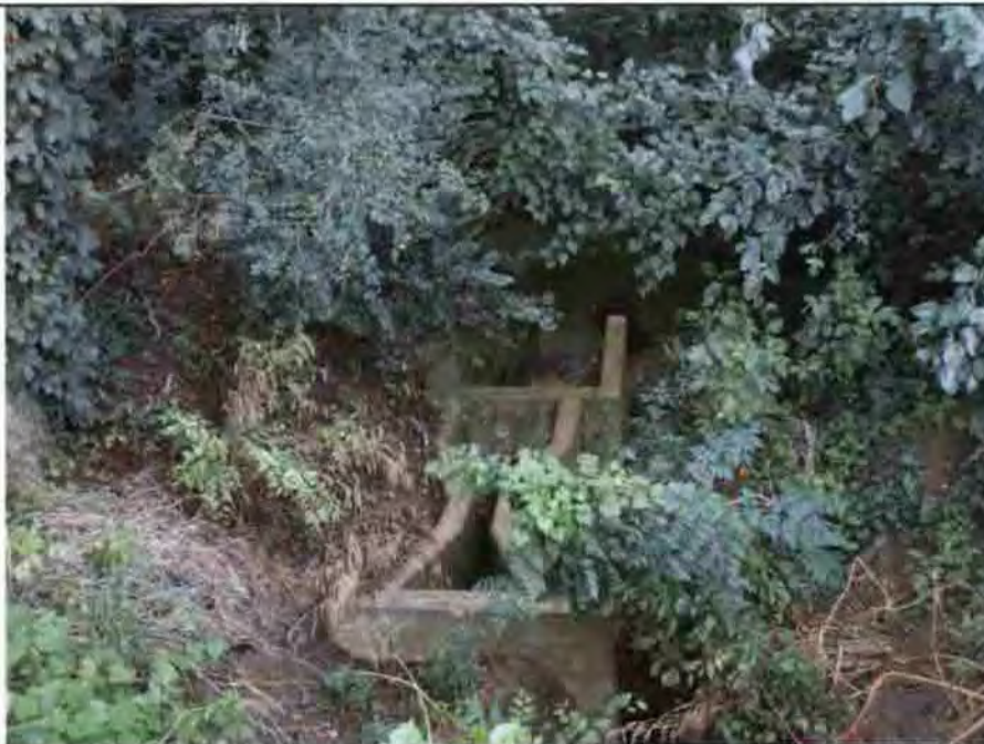
Emergency overflow outfall at weir of former discharge point. Discharge was unpermitted and went to Cottonwood Creek.
