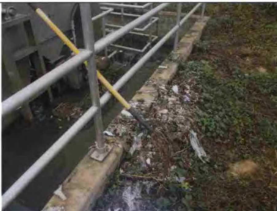
Pile of grit observed on the ground by the bar screen.
