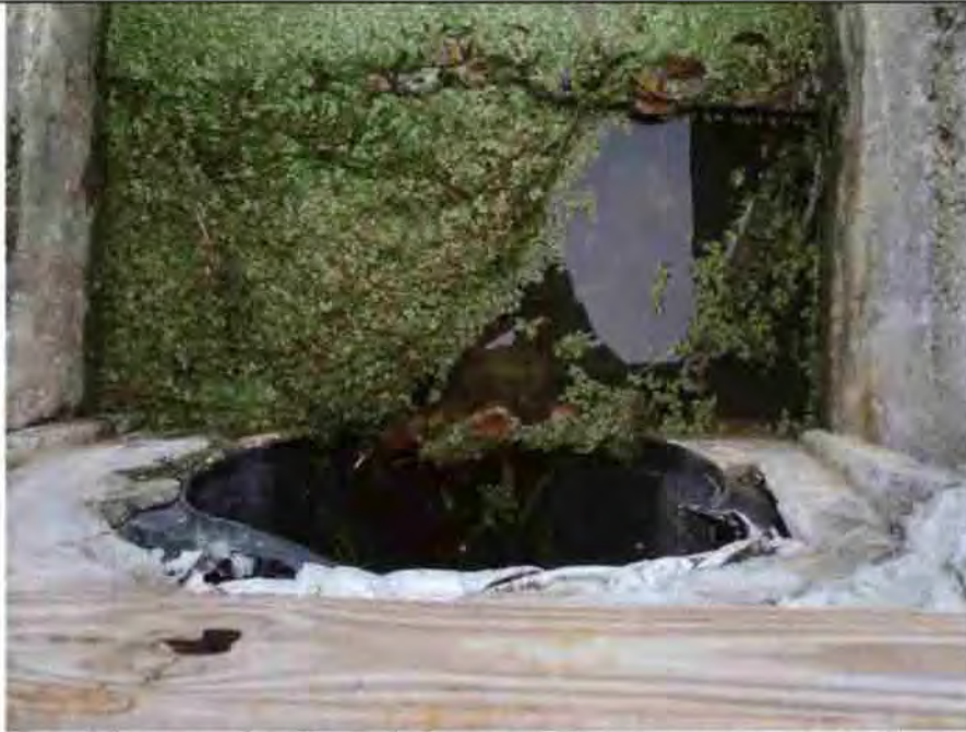
Emergency overflow outfall constructed at a former discharge point. Discharge was unpermitted and went to Cottonwood Creek.
