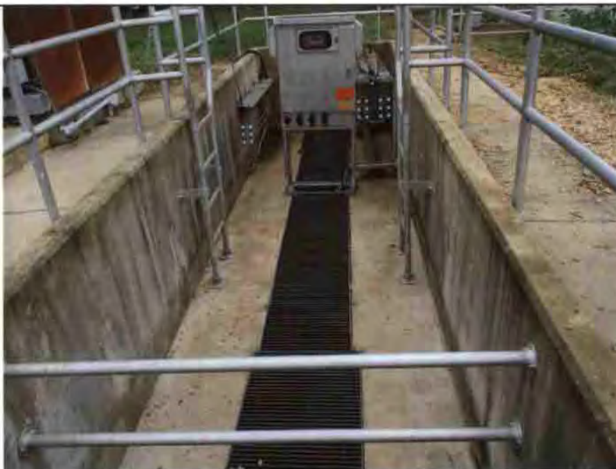
UV disinfection system in place but not operating at the time of the inspection.
