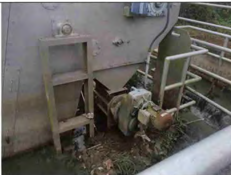
Flooding observed in influent pump and bar screen station. Bar screen motor was damaged.
