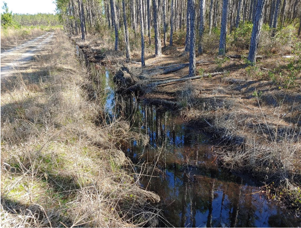
Photo 9. Trail road ditch in the eastern portion of the site.
