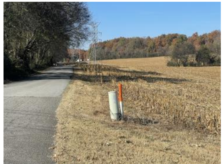
Photo 12 View of electrical components
