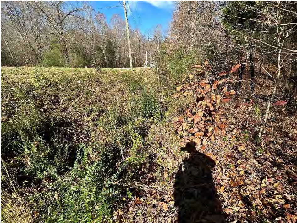
Photo 6: Looking north from N35.724894°, W84.367150° showing the location that WWC 1 flows into the drainage ditch along Carding Machine Road.
