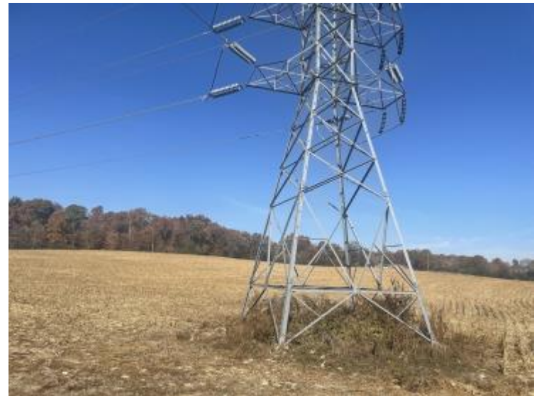
Photo 16 View of transmission lines south of the site
