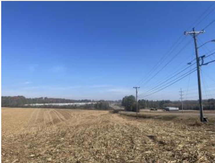
Photo 9 View of the site and pole-mounted transformer facing northeast
