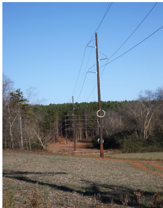
Figure 2.4-1. COR-TEN Monopole Structure with Horizontal Post Insulators
