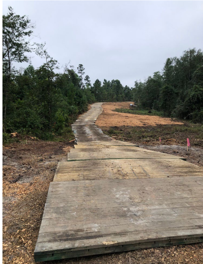
Figure 2.4-3. Timber Mats Placed During Transmission Line Construction.
