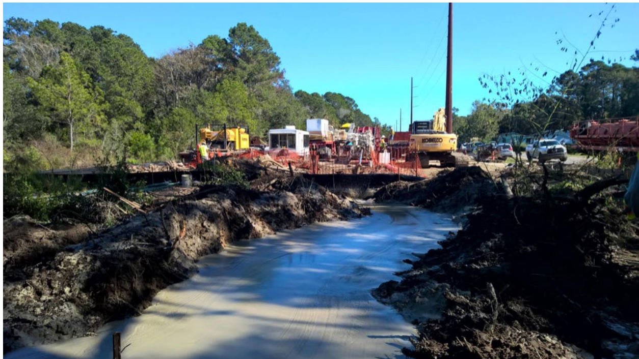
Figure 2.4-2. HDD Drilling Exit Location with the Drilling Fluid Pit in the Foreground
