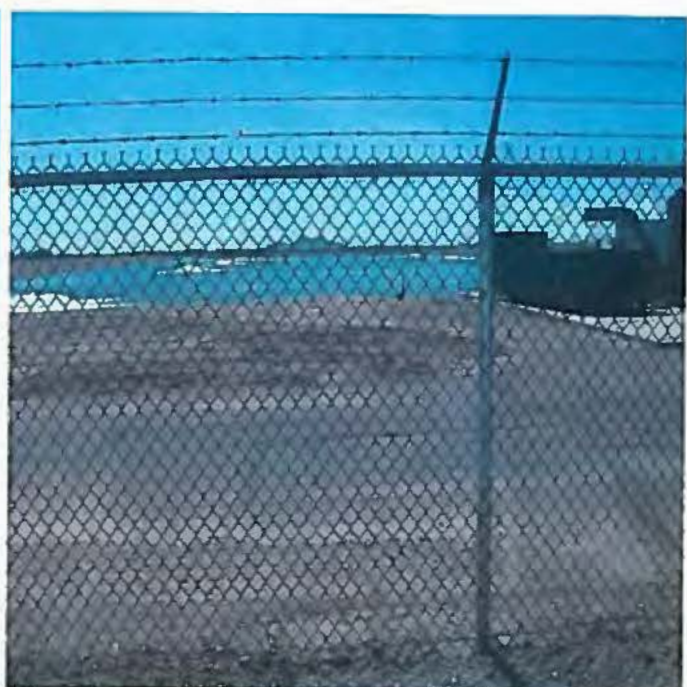
Chander Wastewater Treatment Plant is located north of the proposed project site.
