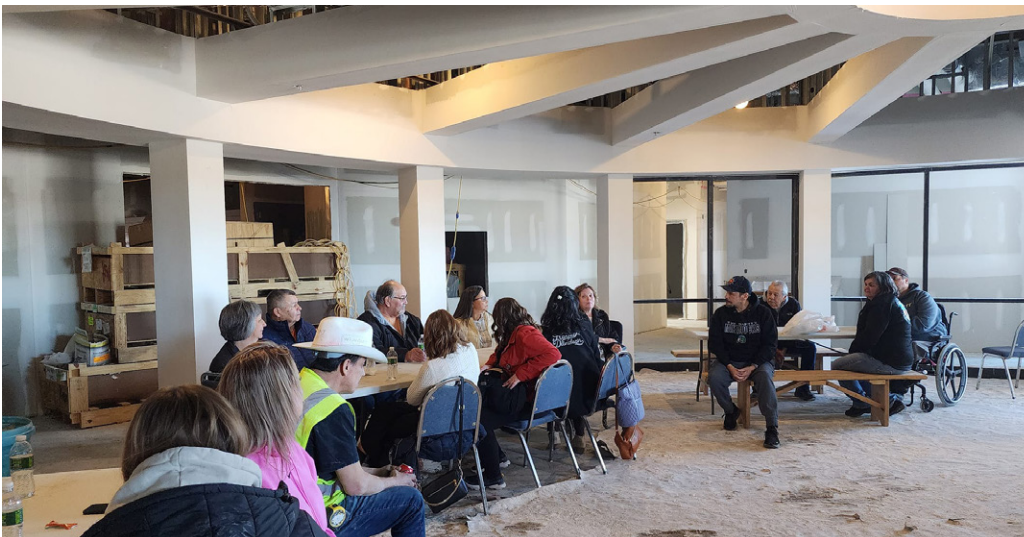
Turtle Mountain Recovery Center during construction.
