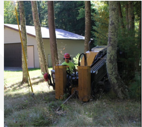
Directional Boring in a sensitive area
