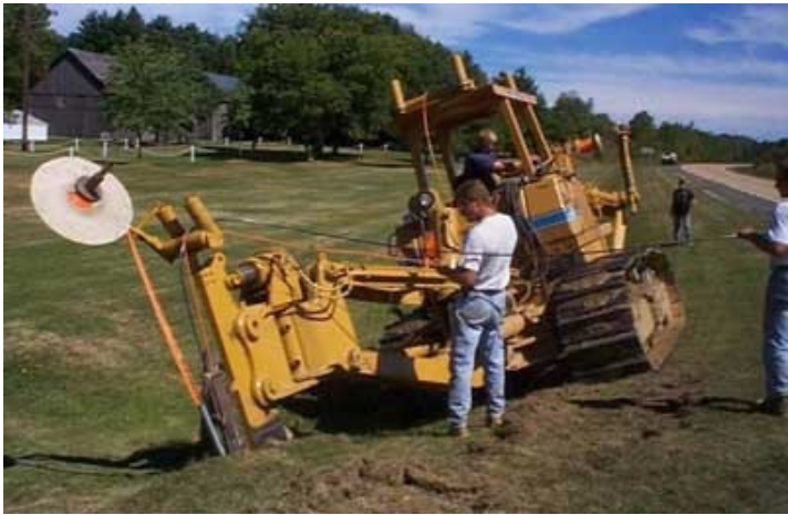
Plowing Method of Installation
