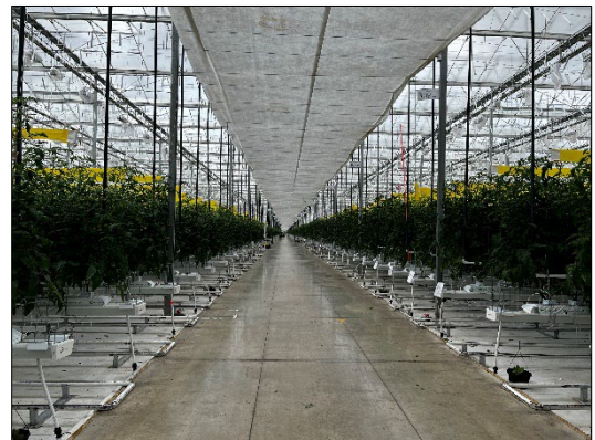
New high-pressure sodium and LED lighting overhead provide "sunshine" for a new tomato crop in Mucci Farms' 75-acre greenhouse in Huron, Ohio. USDA
