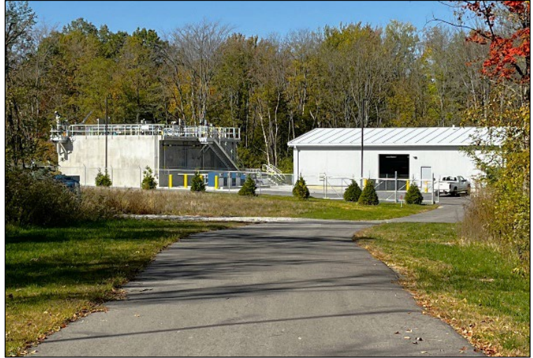
Newtonsville’s new wastewater treatment facility occupies a small footprint and features the single batch reactor (SBR) on the left, and disinfecting building. USDA Photo.
