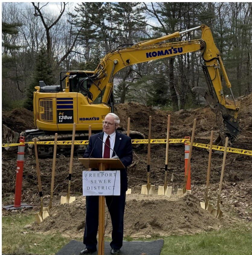
State Director John Butera highlights USDA Rural Development's investment in Freeport's upgraded wastewater system, reducing sanitary concerns and boosting economic development.
