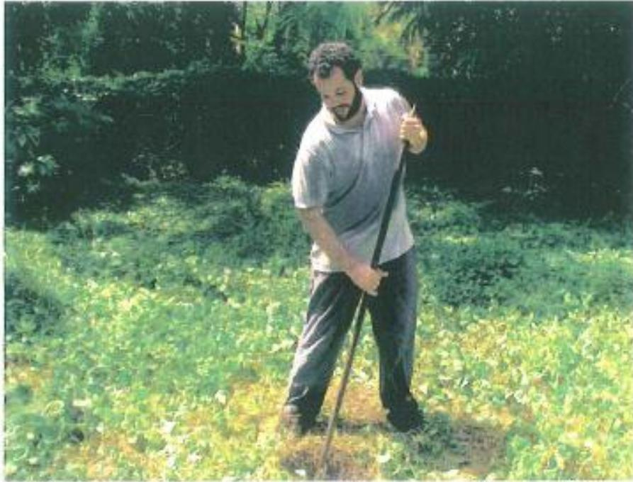
**Photo 6.** Test pit excavation using a digging bar. Looking west.
