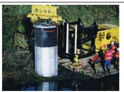
Graphic 2: Vibratory Hammer Installing Caisson
