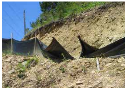
Incorrect Use of Silt Fence
