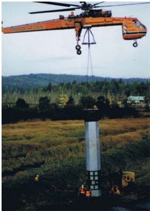
Photograph 1: Helicopter Transporting Steel Caisson to Construction Site
