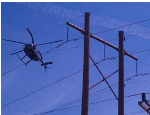
Photograph 4: Helicopter Stringing Wire
