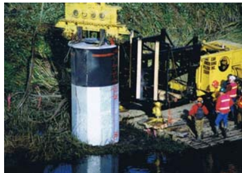
Photograph 3: Vibratory Hammer Installing Caisson
