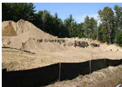
Proper Use of Silt Fence
