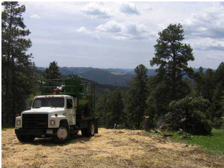
Temporary access (low-traffic) using mulch
