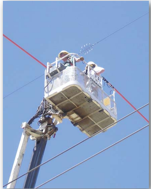
Installation of swan flight diverters (above)
