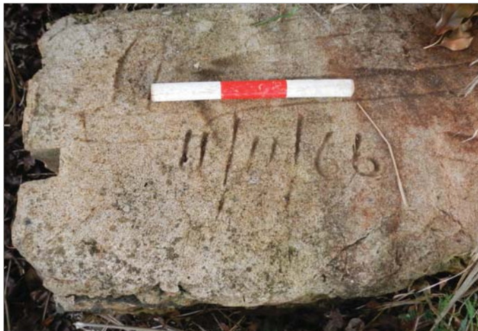
Figure 23: Detail photograph of the “11/11/66” date inscription on a site 50-30-08-2160, Ditch 1 sluce gate fitting, looking down. Note the grooves at the left of the frame for the sluce gate boards. Figure 22 depicts an expanded view of this sluce gate fitting. The scale is in decimeters.
