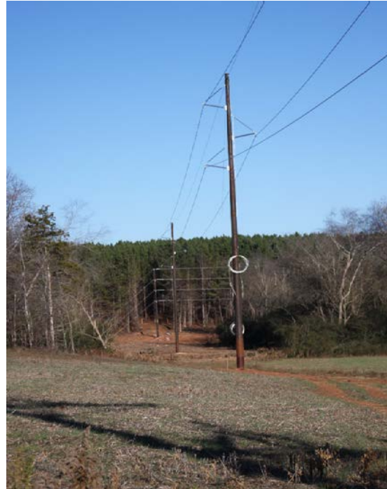
Photograph 1: COR-TEN Single Pole Structure with Horizontal Post Insulators
