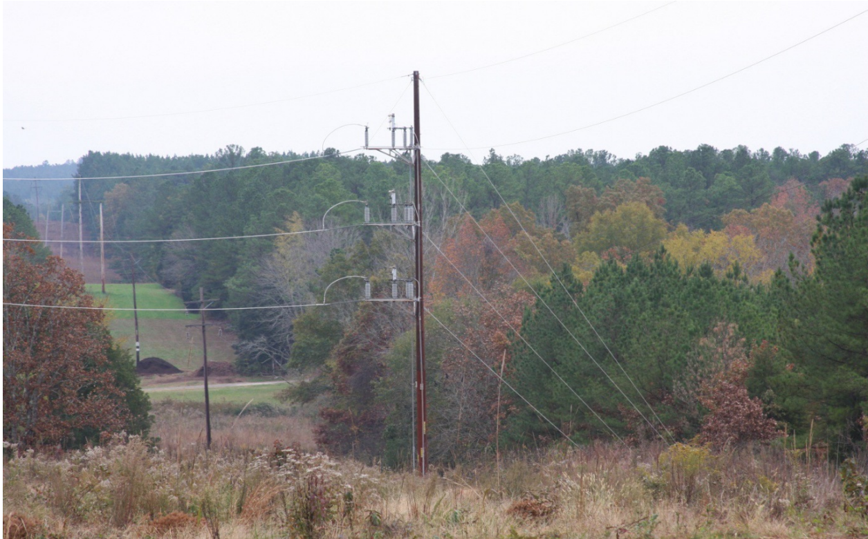
Figure 4-6: Typical Line Switch
