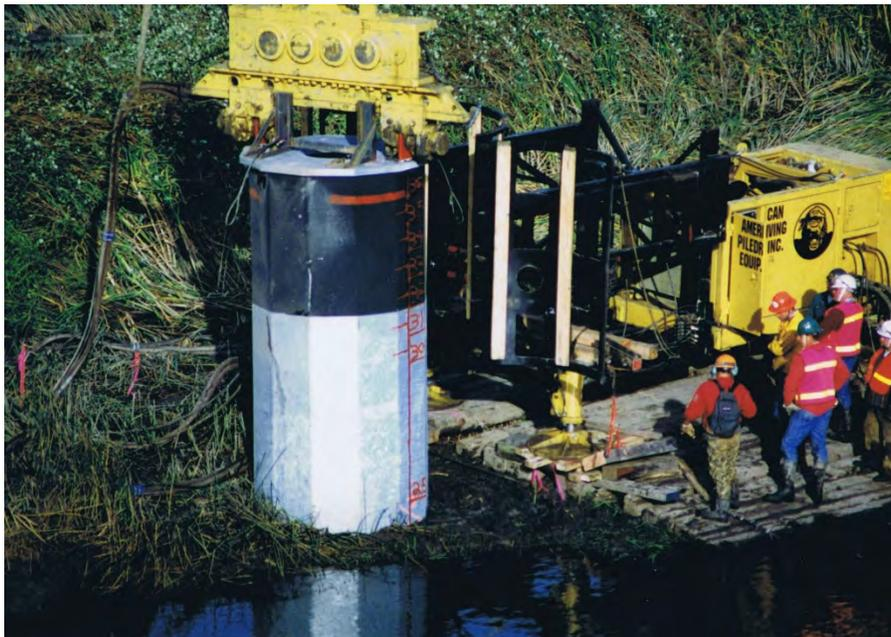
**Helicopter Based Vibratory Caisson and Hammer Unit**
