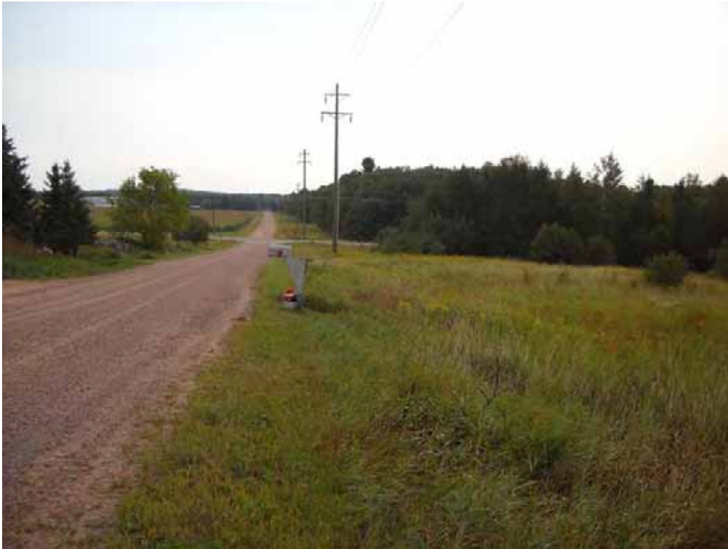
Photo 5. View of Kempton Road north of US212 near Bridge Creek Substation looking south.
