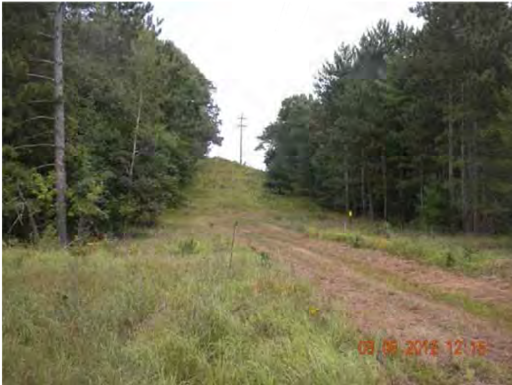
Photo 4. View from Kempton Road approximately 0.7 mile north of County Road RR looking northeast at the Project ROW.
