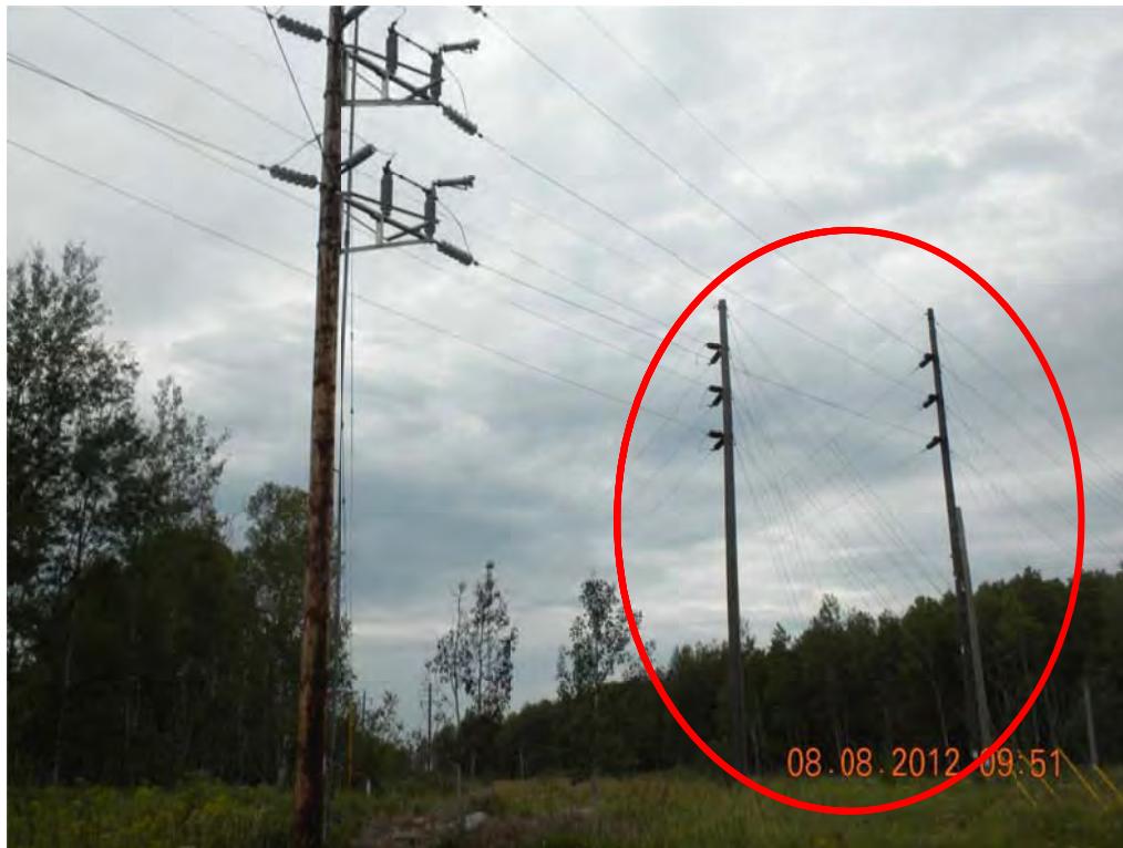
Photo 5. View of switch structures on the southwest corner of County Line Road and Sterling Avenue near Lublin Substation.
