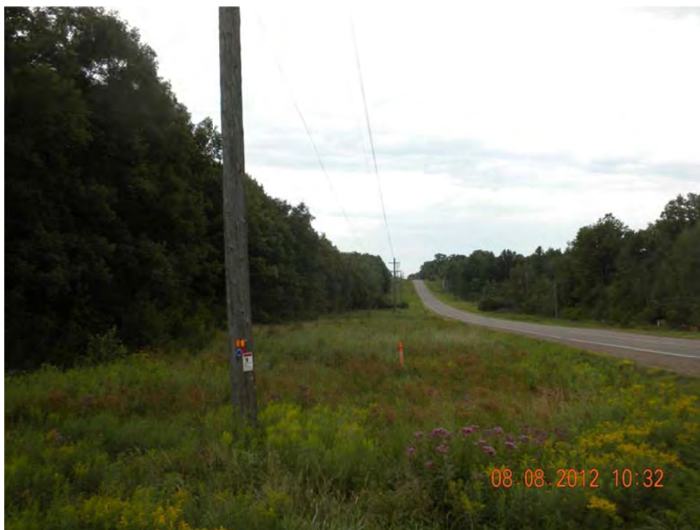
Photo 2. View from Starks Road looking south at the Project ROW along the east side of County Road M.
