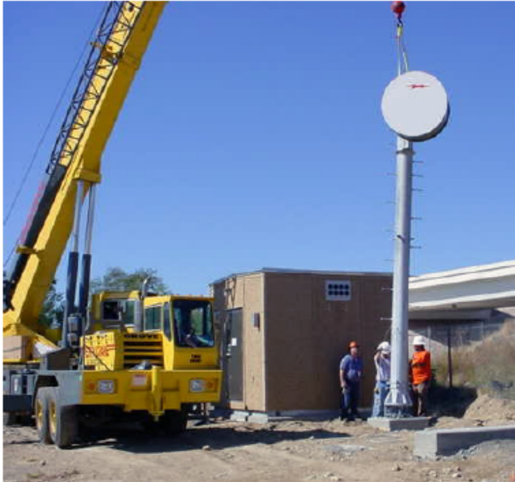
Figure 2-12. Final construction of a microwave tower. Source: Power and Communication Contractors Association
