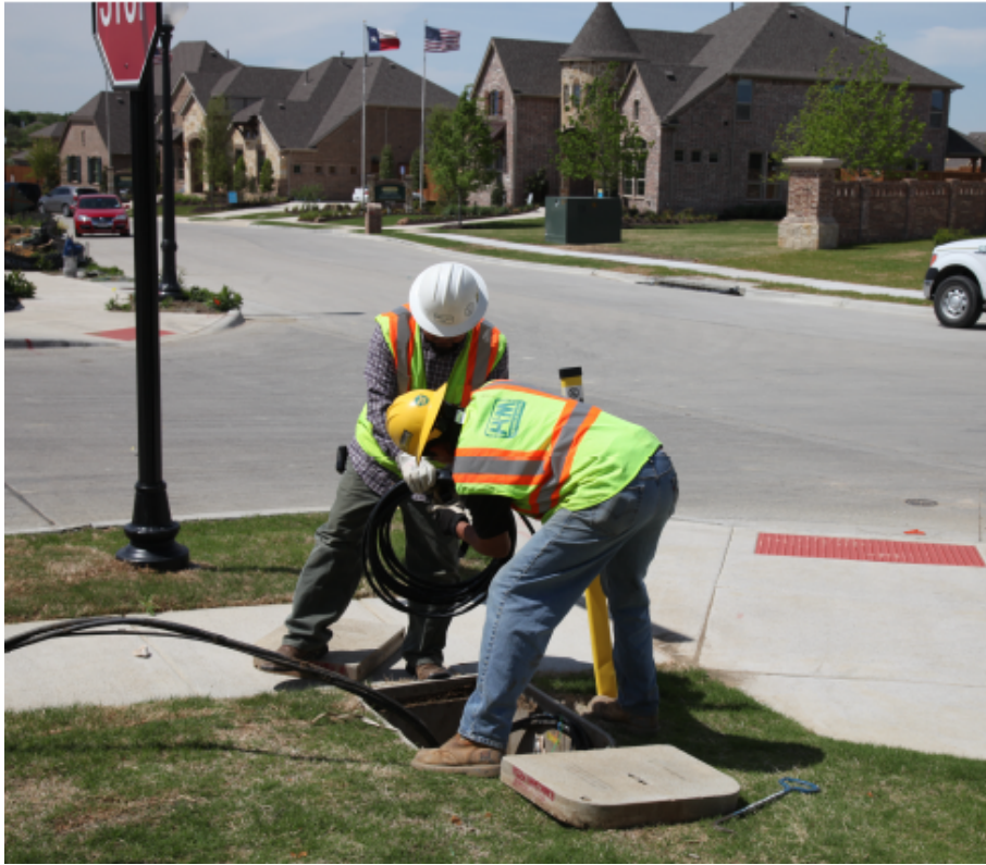
Figure 2-8. A handhole in a suburban neighborhood. Source: Power and Communication Contractors Association
